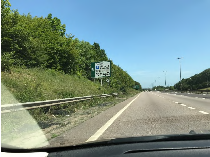
A120 (From M11 North/A120 Interchange)
